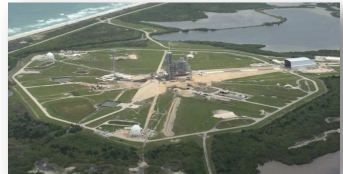
LC-39A with Renovations in Progress
